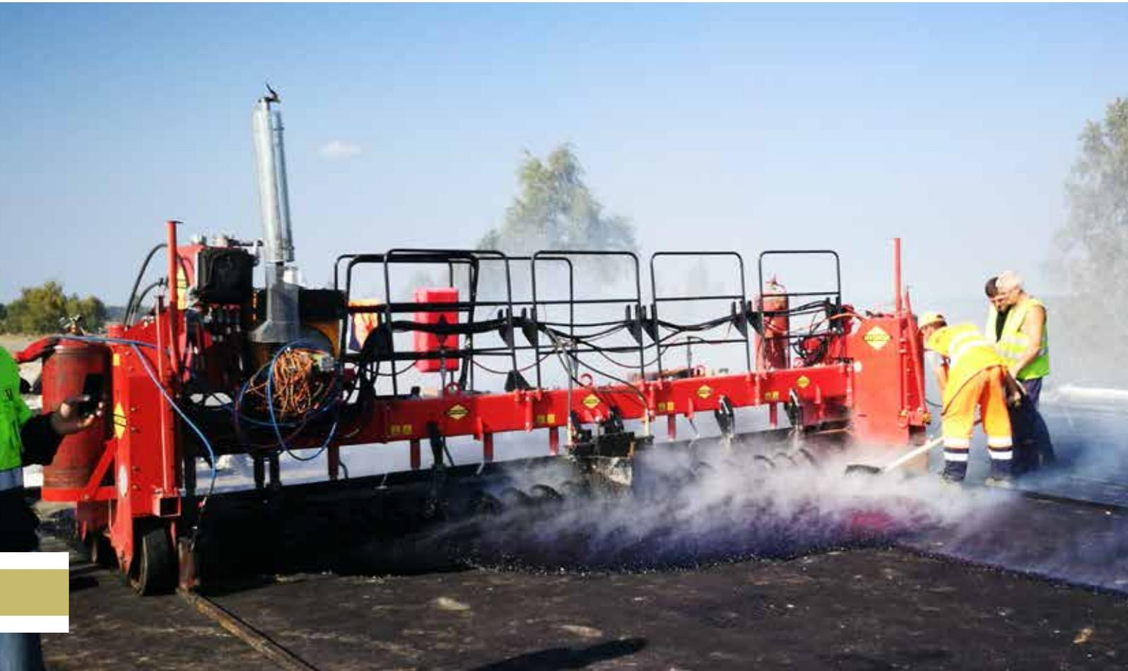
**Mastic asphalt finishers HYDROG RAL-5500 and RAL-7500 are used for machine spreading, levelling and compaction of layers of mastic asphalt with a heated bar (blade) during the execution of**
